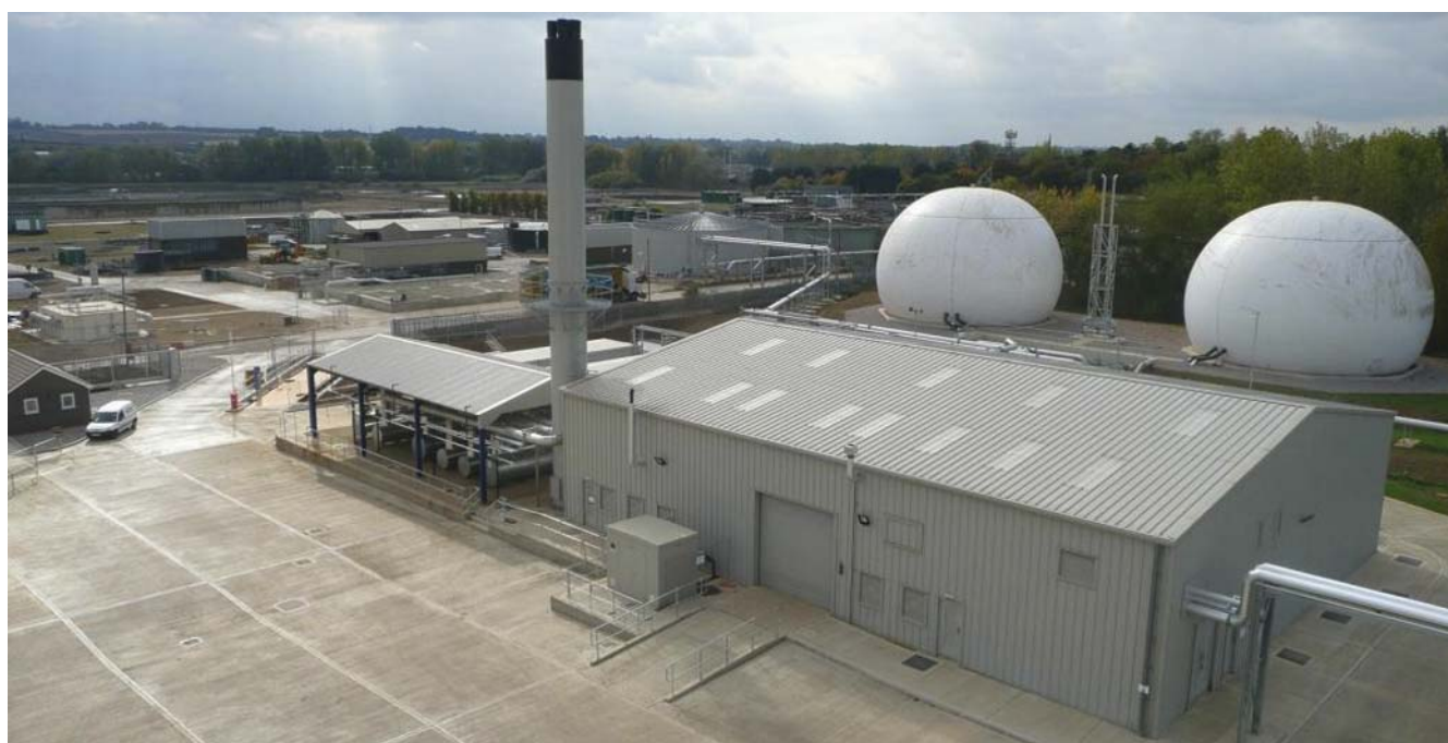
Great Billing - Heating building, gas holders, waste heat boilers and digesters from the top of the Monsal EEH plant
