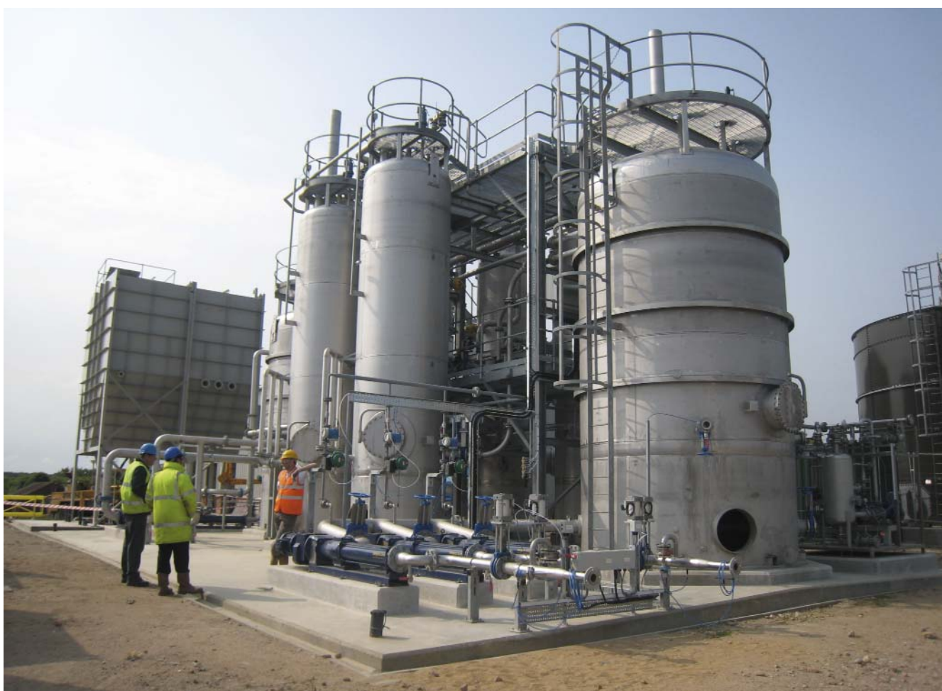
Whitlingham – Cambi thermal hydrolysis plant under construction
