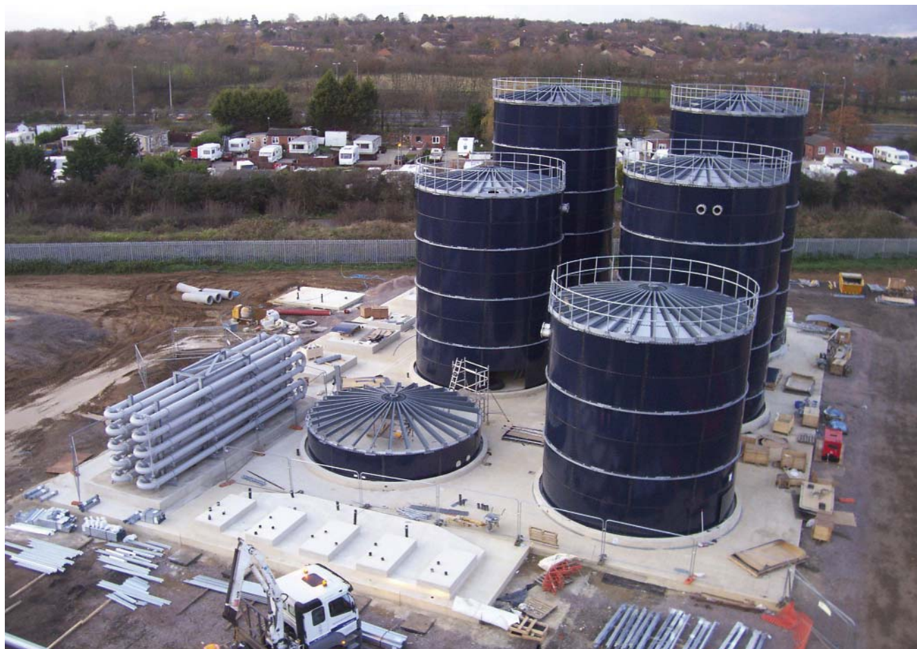
Great Billing – Monsal EEH biological hydrolysis plant under construction
