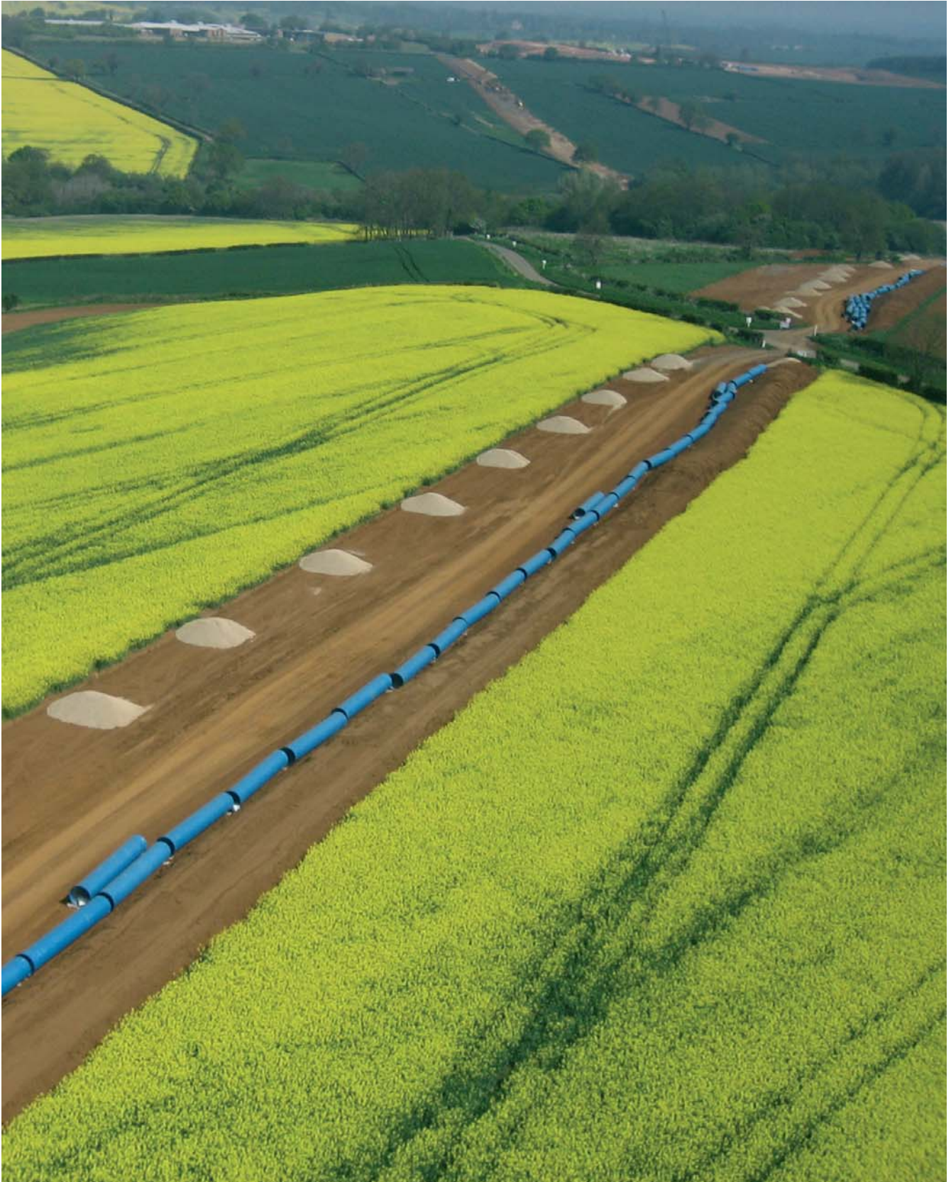
Wing to Beanfield Pipeline
