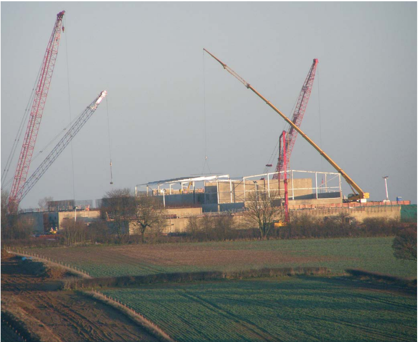
Morcott Water Treatment Works under construction
