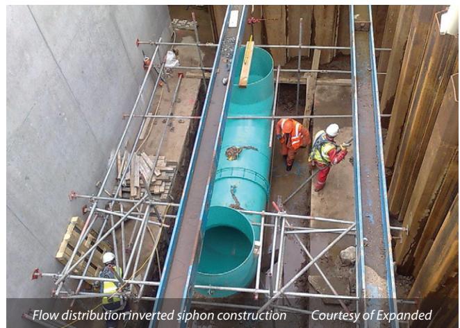
Flow distribution inverted siphon construction Courtesy of Expanded
