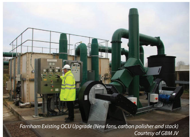
Farnham STW New Air Mixing System to Existing Sludge Import / Buffer Tank - Courtesy of GBM JV
