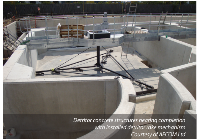
Intermediate shaft between sewer connection/TLLPS. This will ultimately include a baffle wall, developed by Hydrotec Ltd to prevent formation of a standing wave in the tunnel downstream – Courtesy of AECOM Ltd
