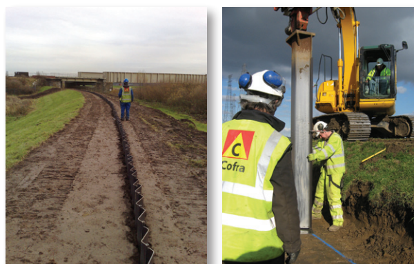
Plastic pile installation at Gainsborough Flood Alleviation Scheme
