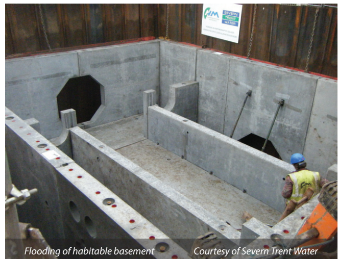
Siphon Riverside CSO under construction Courtesy of NMCNomenca
