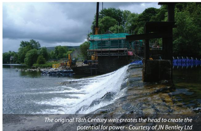
*The original 18th Century weir creates the head to create the potential for power - Courtesy of JN Bentley Ltd*
