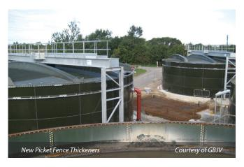
**Thickeners:** The provision of an additional 2 (No.) 15m diameter Picket Fence Thickeners from MWH Treatment to supplement the 2 (No.) existing Thickeners.
