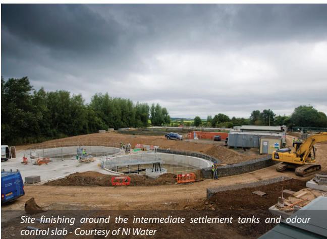
New thickened sludge holding tank filling for water test Courtesy of NI Water
