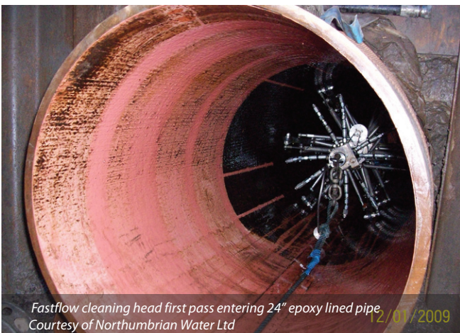
900mm Allerburn cross connection Courtesy of Northumbrian Water Ltd
