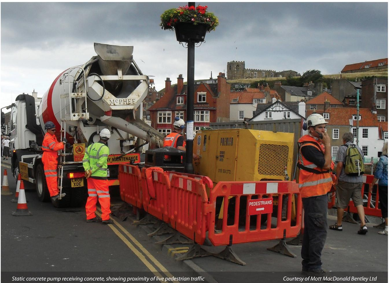
Static concrete pump receiving concrete, showing proximity of live pedestrian traffic
