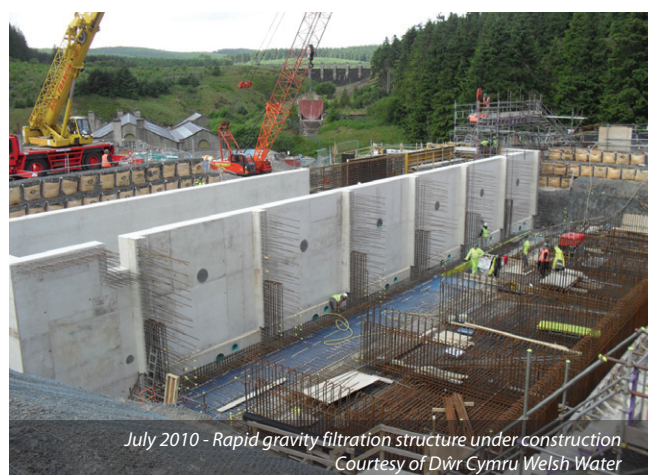
June 2010 - Rapid gravity filtration structure under construction Courtesy of Dŵr Cymru Welsh Water
