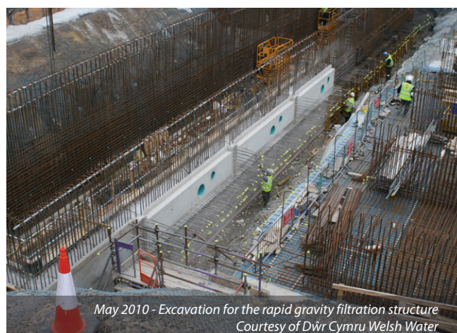
April 2010 - Excavation for the rapid gravity filtration structure Courtesy of Dŵr Cymru Welsh Water
