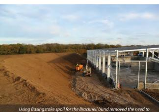
Using Basingstoke spoil for the Bracknell bund removed the need to import 20,000 tonnes of virgin material - Courtesy of Black & Veatch
