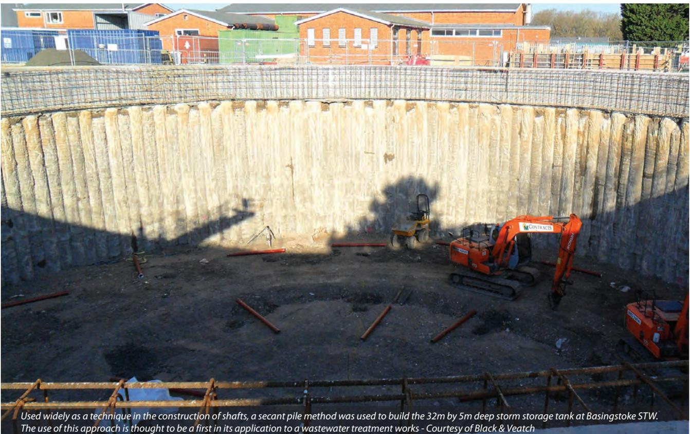
*Used widely as a technique in the construction of shafts, a secant pile method was used to build the 32m by 5m deep storm storage tank at Basingstoke STW. The use of this approach is thought to be a first in its application to a wastewater treatment works - Courtesy of Black & Veatch*
