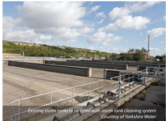
Existing final settlement tanks to be refurbished and bridges removed and replaced with new - Courtesy of Yorkshire Water
