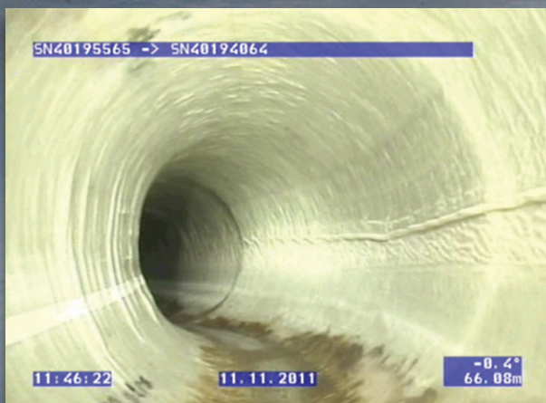
CCTV footage of CIPP lining Courtesy of Dŵr Cymru Welsh Water
