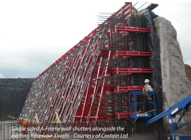
Reinforced Concrete Works: the base slab and valve chamber walls already in place with the reservoir walls and columns mid construction Courtesy of Costain Ltd
