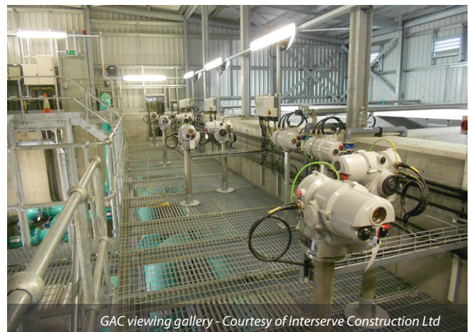
GAC building - Courtesy of Interserve Construction Ltd
