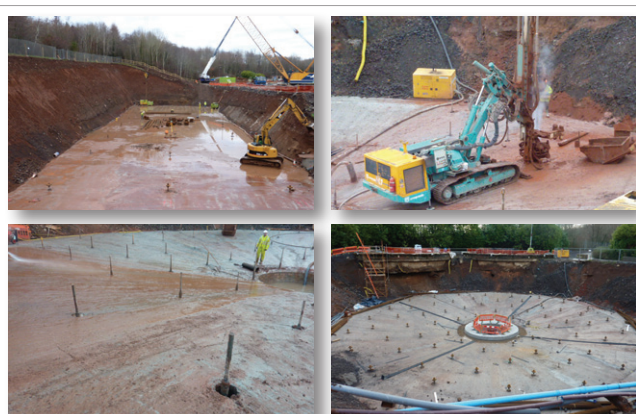
Tank excavation and rock anchors - Courtesy of NI Water
