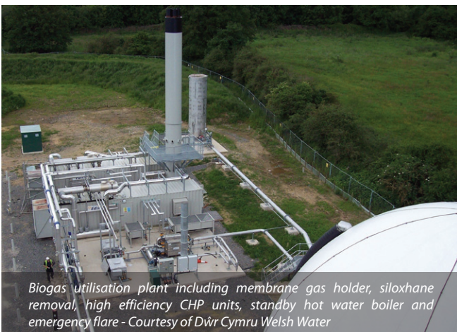
New sludge digestion plant including raw sludge storage, thickening, thickened sludge buffer tank, anaerobic digesters, odour control, and main control building - Courtesy of Dŵr Cymru Welsh Water
