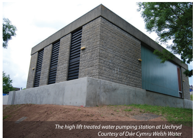
New control building at Llechryd Pumping Station Courtesy of Dŵr Cymru Welsh Water
