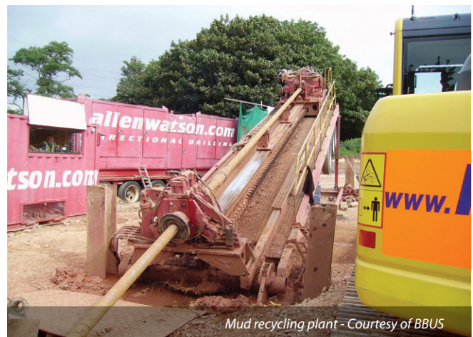
Horizontal directional drilling rig - Courtesy of BBUS
