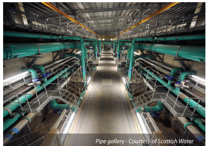
Construction is underway - Courtesy of Scottish Water
