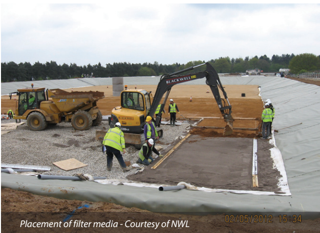
Filtrate drainage and stone layer placement - Courtesy of NWL
