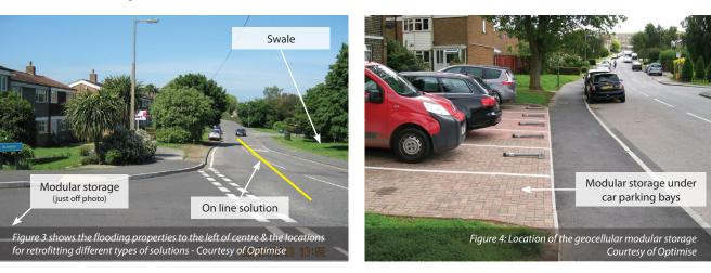
An important element of the swale in Rye Meads was to understand how it would work. It would only be operational to 'peak lop' significant rainfall.
