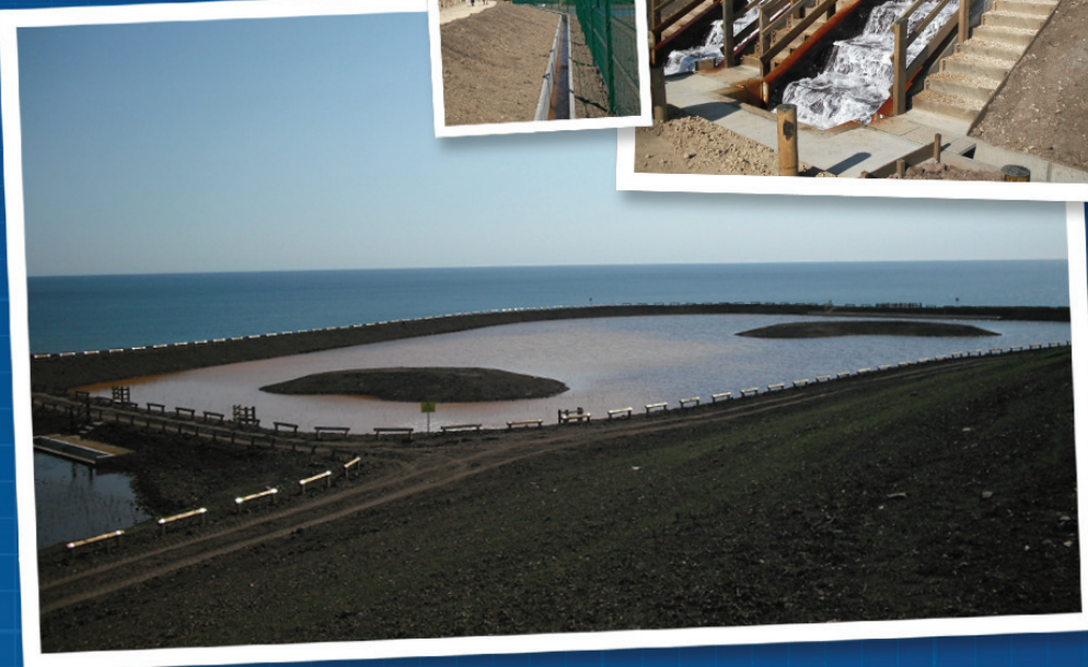
Horden Passive Minewater Treatment Scheme, County Durham
