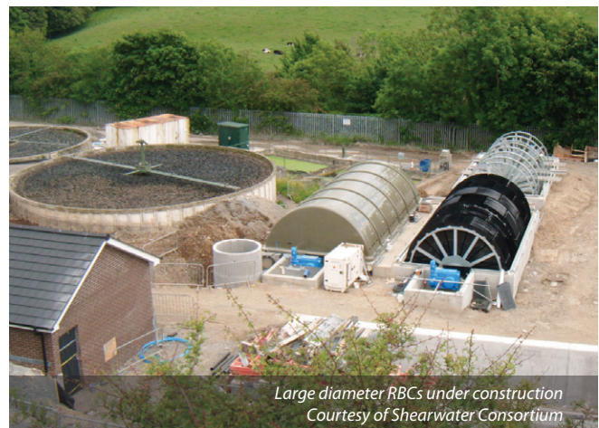
Keady WwTW - Start of work - December 2010 Courtesy of Shearwater Consortium
