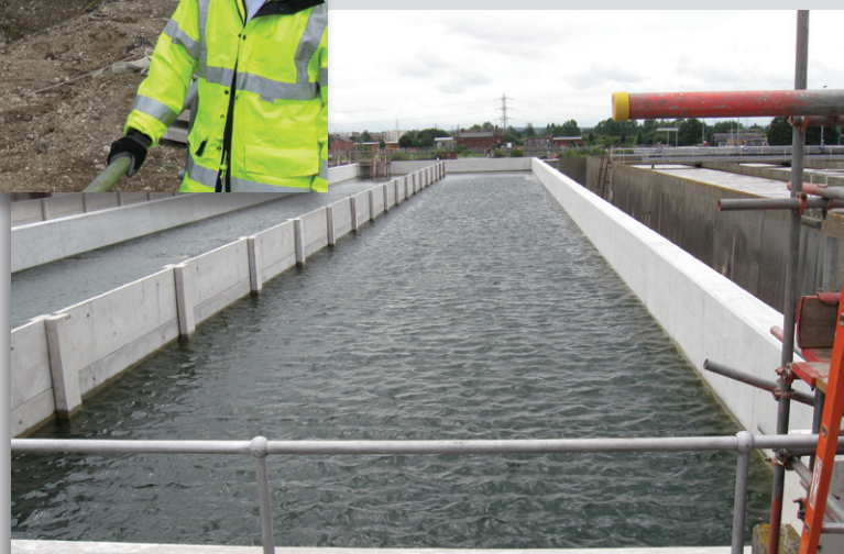
New Aeration Tank undergoing water test Courtesy of Mott MacDonald
