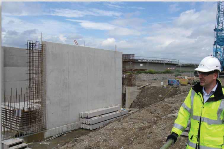
Aeration tank under construction Courtesy of Mott MacDonald
