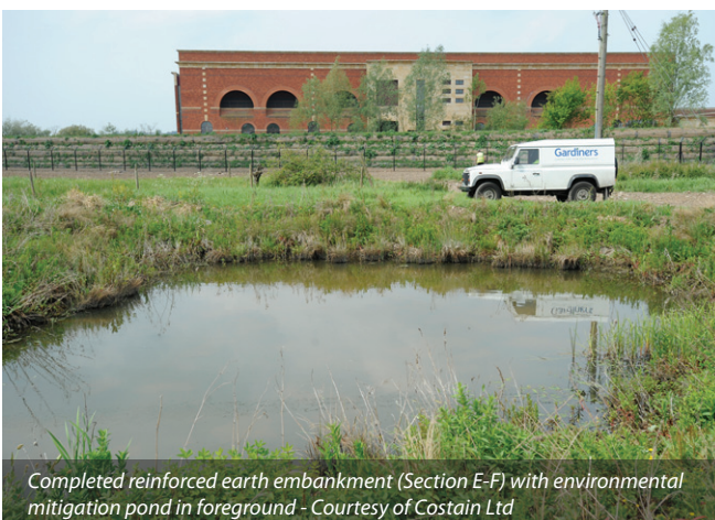
Section G-H brick clad RC wall looking south alignment specified to avoid existing services - Courtesy of Costain Ltd
