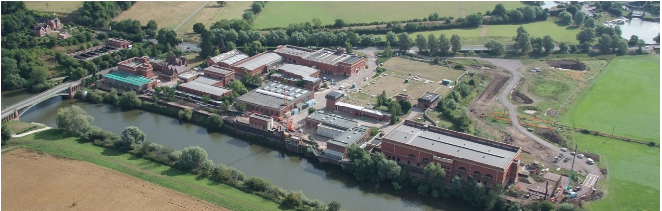
Mythe WTW looking from the west with the River Sever in the foreground - Courtesy of Severn Trent Water
