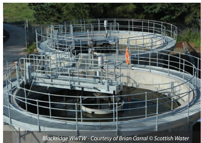
Torphichen WwTW - Courtesy of Brian Carral © Scottish Water
