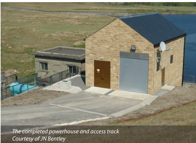
The portal frame structure of the powerhouse was clad with masonry and appropriate roofing materials to give a traditionally-built barn impression - Courtesy of JN Bentley
