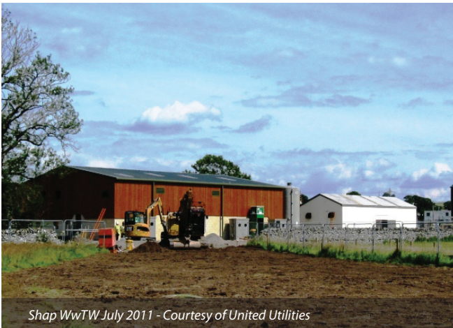
March 2011 - Construction of MBR tanks - Courtesy of United Utilities
