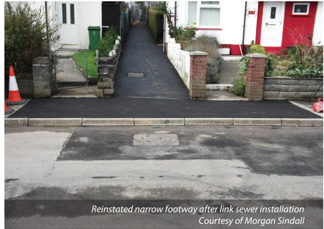
Reinstated narrow footway after link sewer installation
