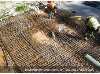
The contact tank was of a reinforced concrete structure of  $16m \times 15m \times 4m$ . The walls of the structure had been designed at 350mm thick to allow the structure to be water retaining. The steel rebar used within the reinforced structure was also designed at the European coding of 51xD.
