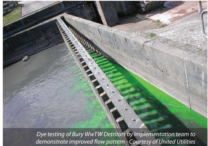
*Dye testing of Bury WwTW Detritors by Implementation team to demonstrate improved flow pattern - Courtesy of United Utilities*
