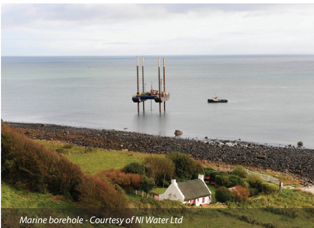
Whitehead New Pumping Station - Courtesy of NI Water Ltd
