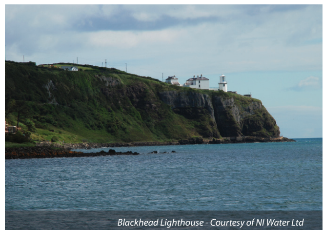
Whitehead New Pumping Station (from viewing platform facing south) Courtesy of NI Water Ltd - Courtesy of NI Water Ltd
