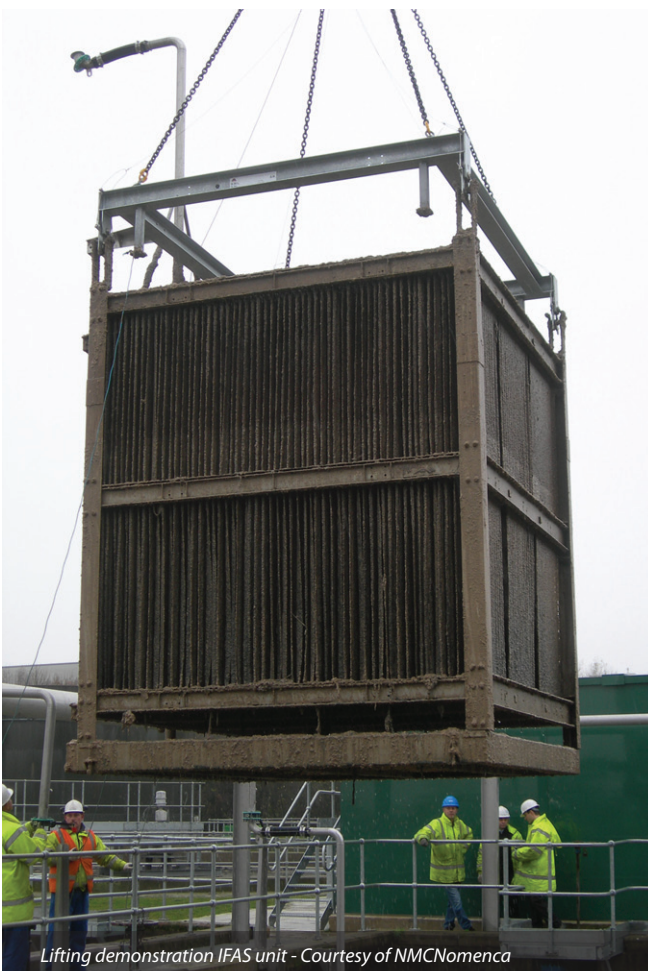
IFAS unit during installation - Courtesy of NMCNomenca
