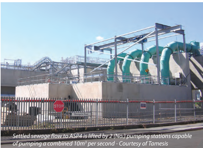
ASP4 RAS/settled sludge pumping station - Courtesy of Thames
