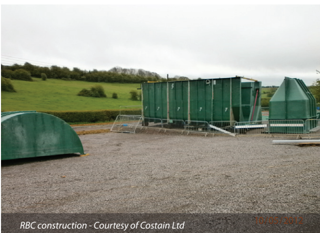
Rotor/media pack installation (aerated reed bed 1 foreground) Courtesy of Costain Ltd
