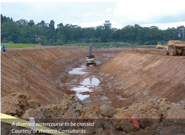
The site with one of the diverted watercourses Courtesy of Waterco Consultants
