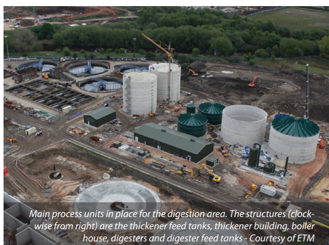
Plant under construction - Courtesy of ETM
