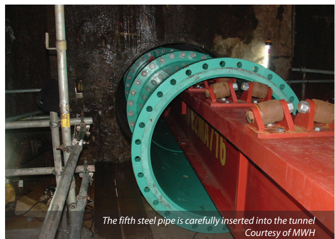
The site set up needed careful consideration within the limited space
