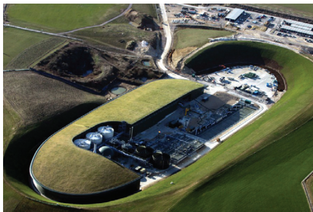
Peacehaven WwTW - Courtesy of Southern Water
