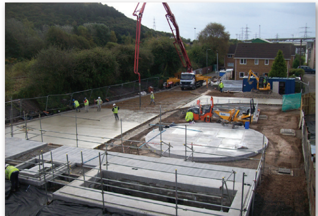
Pumping Station road pour - Courtesy of Morgan Sindall plc
