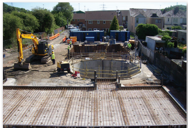
Preparation of kiosk baseslab - Courtesy of Morgan Sindall plc
