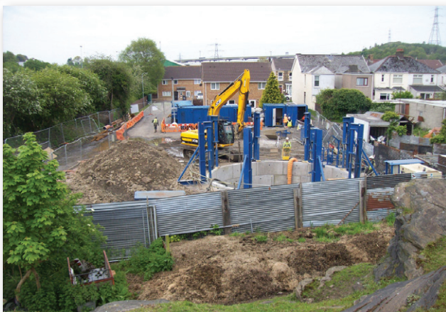
Sinking of stormwater shaft - Courtesy of Morgan Sindall plc
