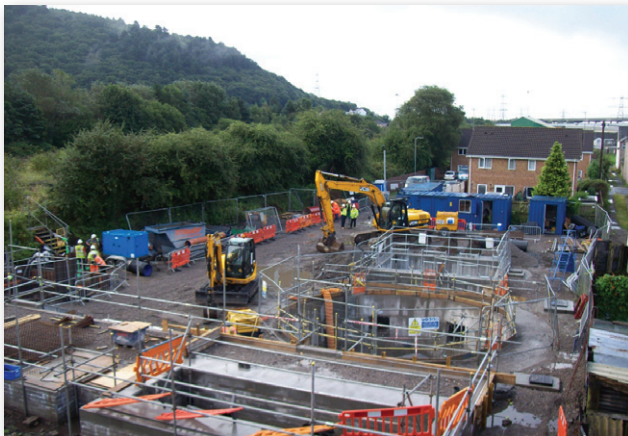
Shaft and kiosk base constructed - Courtesy of Morgan Sindall plc
