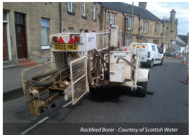
PU lining spin up prior to lining - Courtesy of Scottish Water
