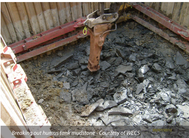
SAF tank contract lift - Courtesy of WECS
