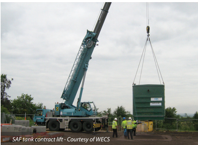
Placing of primary tank - Courtesy of WECS
