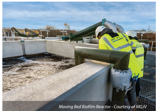
Packaged inlet works - Courtesy of MGJV
