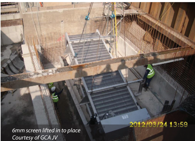
Temporary access bridge lifted into position on precast abutments Courtesy of GCA JV
