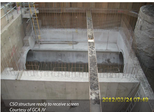
Under construction adjacent to Peak Forest Canal Courtesy of GCA JV
