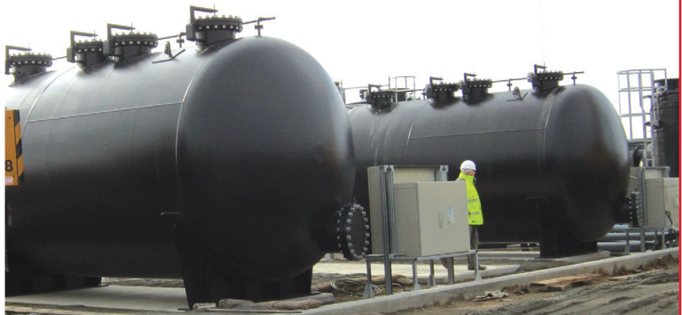
GAC & Pressure Filter Vessels used in Guernsey Airport Water Treatment Facility DESIGNED & MANUFACTURED BY PRESSVESS
